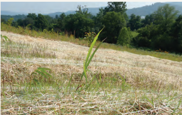
Seedlings from a steep slope mix poking through an erosion control blanket.
