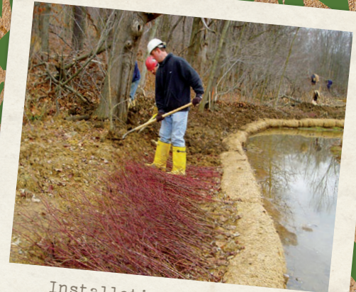
Installation of a brush mattress.
