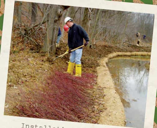
Installation of a brush mattress.
